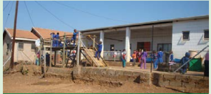
New fencing constructed at God's Little Lambs
